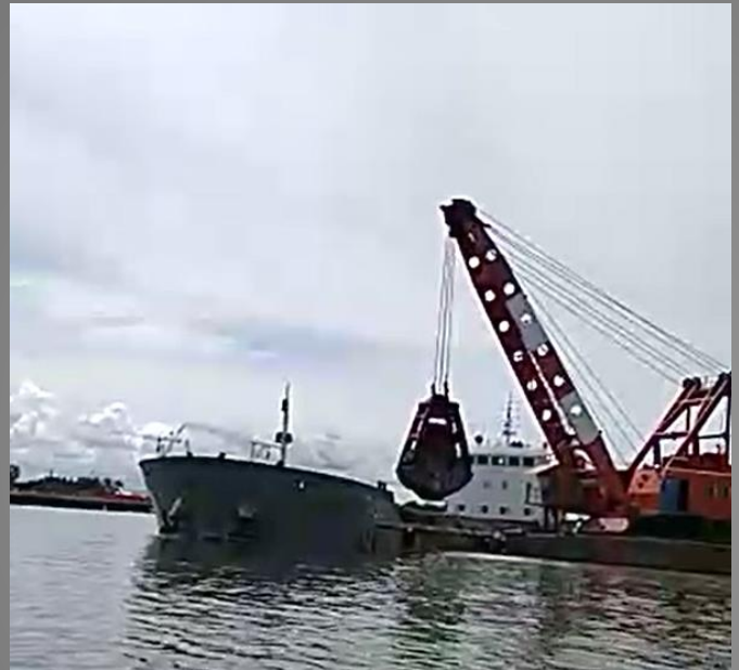
Split barge GJ 502 and clamshel dredger GJ 701 undertake capital dredging for port basin and access channel.
