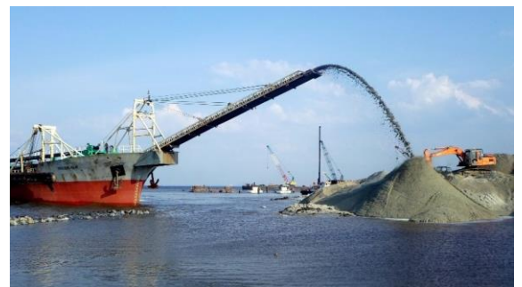
From top: Trailing Suction Dredger GJ 801 delivers materials for reclamation use; Trailing Suction Dredger Sukabumi Maju
